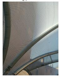
A lateral enclosure is also planned to protect against inclement weather. The vertical canvases are removable and are made with an FT381 mesh fabric from the Ferrari company.
